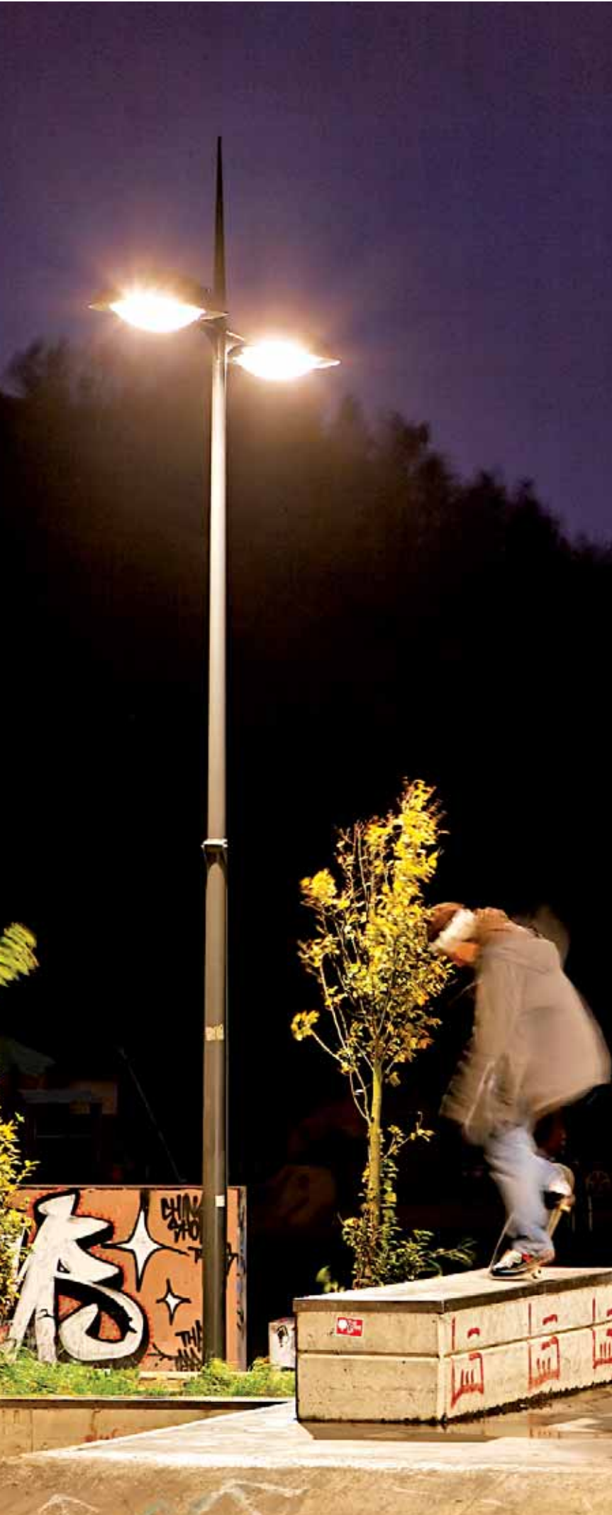
Rio with dished polycarbonate glazing Central Forest Park, Stoke-on-Trent
